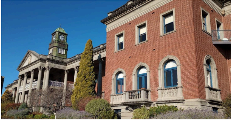
The original 1893 Heritage building.
